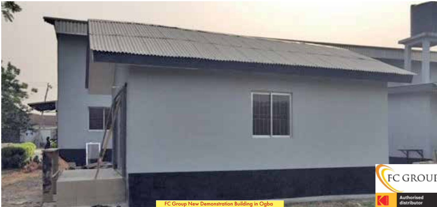
FC Group New Demonstration Building in Ogba
