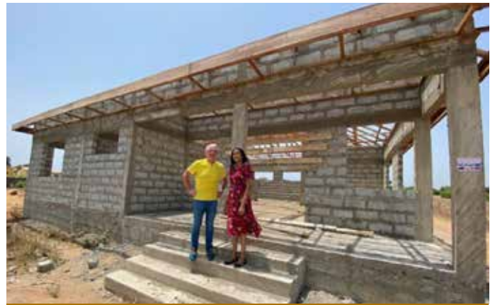
Fenton on site roofed Library Project with Zeena (c) FC Group.
